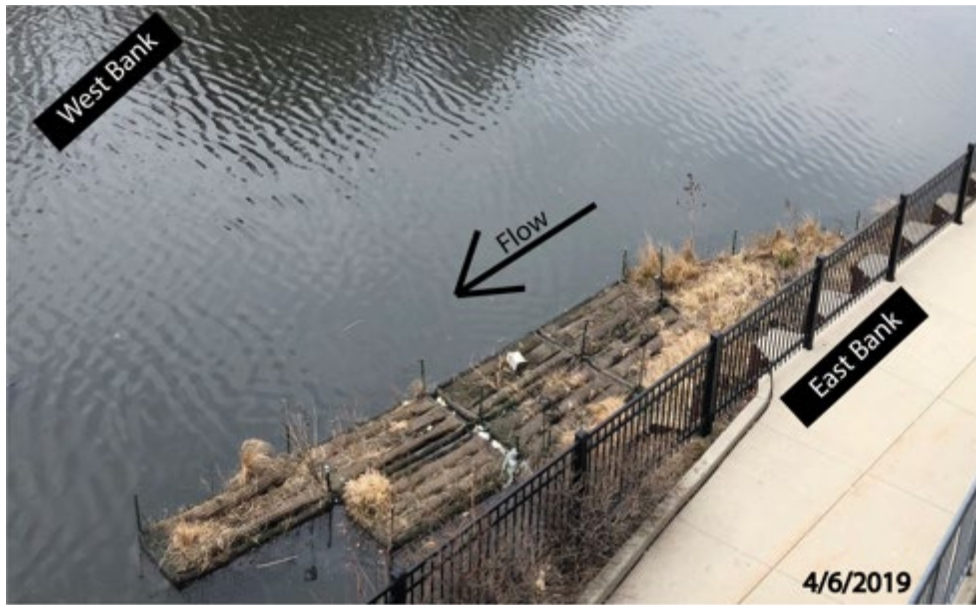
Figure 3: Floating substrate made of coconut husk used for planting on the gardens.
