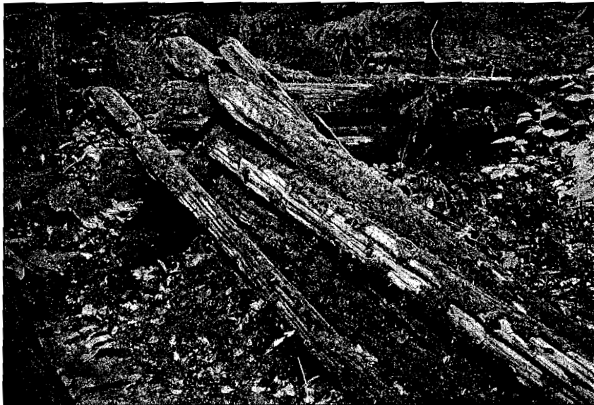
Figure 9. Structure B, southeast corner, looking southwest.
