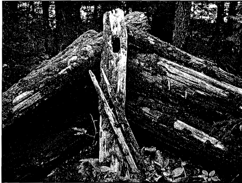
Figure 11. Structure B, southeast corner, looking southeast from inside.
