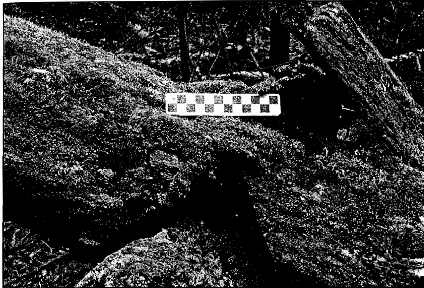
Figure 10. Structure B, southeast corner, notching detail.
